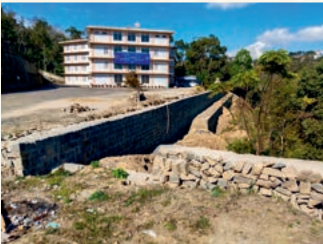
Construction of retaining wall & security fencing below New Directorate Office, Kohima.
