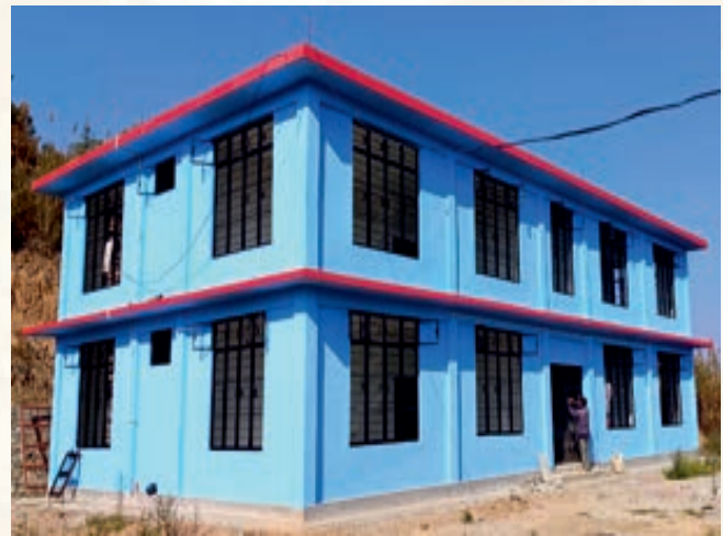
Construction of District Economics & Statistics Office at Noklak.
